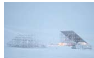
Superstructure for RISR-C.
